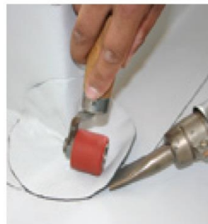
Details for the Treatment of Outside Corner
