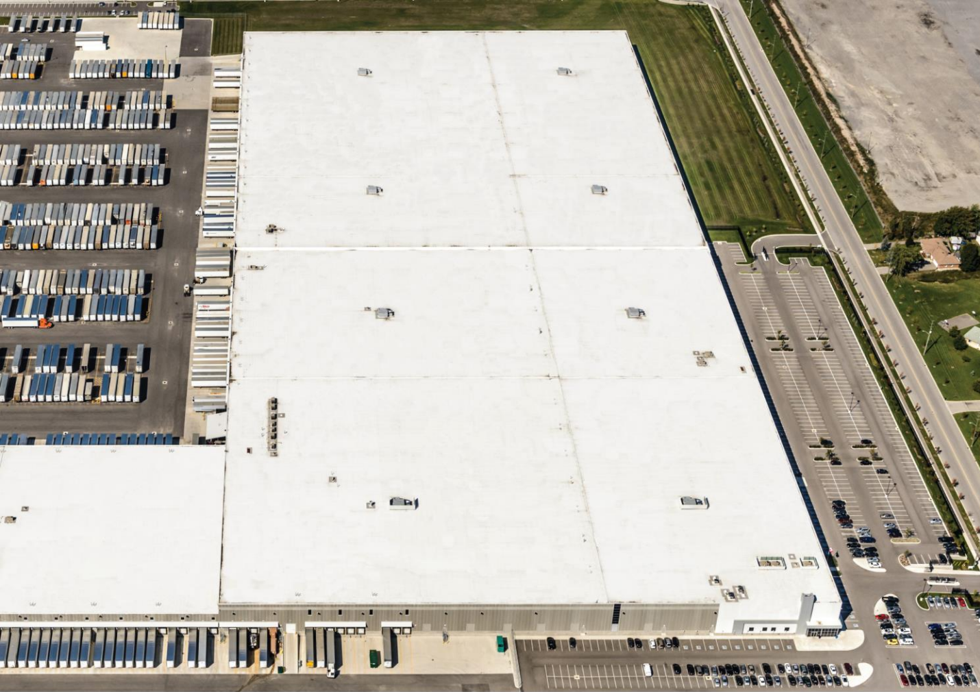
A reflective Sika roofing membrane was selected to cover the 1.3 million square foot Target Distribution Centre in Milton, Ontario
